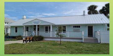
In May, Public Works finished an exciting project, the rebuild and extension of the Community Center's front porch. The new porch is covered in weather-resistant decking and extends west from the original porch's footprint to the side door. The PW team also repainted all of the Community Center's trim in an effort to further beautify the building's exterior.
