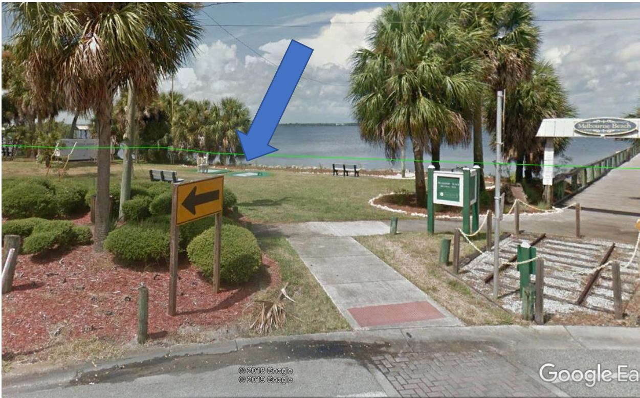
Figure 19 Ryckman Park with Lift Station near Indian River Lagoon (from Google Earth)
