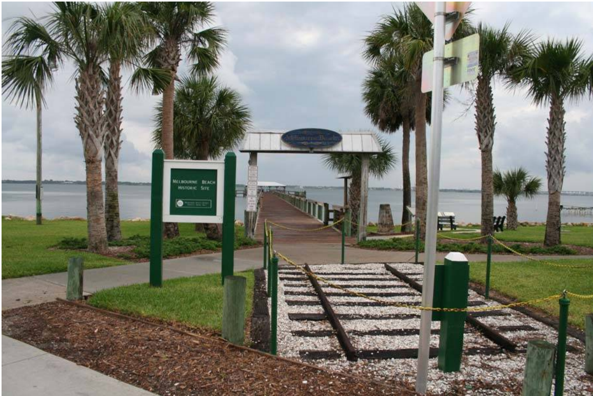
View of Melbourne Beach Pier
