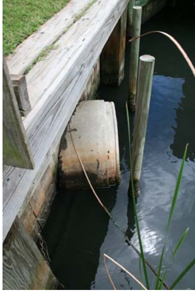
Typical Canal Outfall
