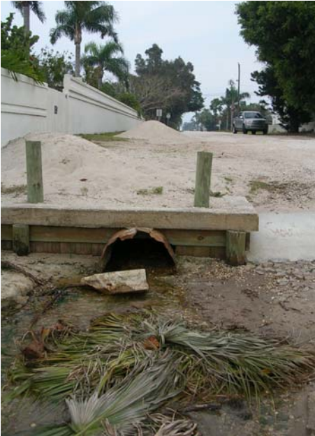
Sixth Avenue Outfall
