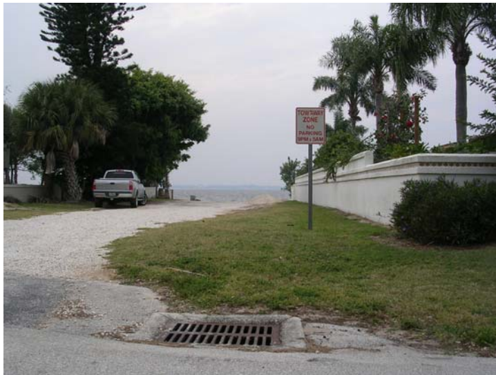
Sixth Avenue Outfall
