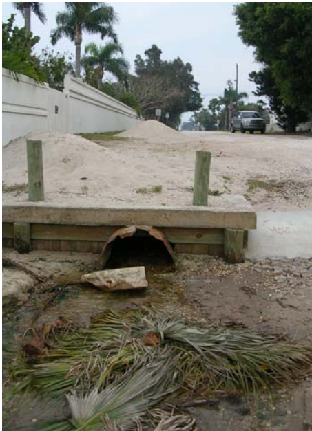
Sixth Avenue Outfall
