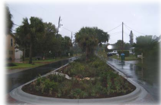
Photo 2 West End of Sunset Boulevard Looking East Post-Construction
