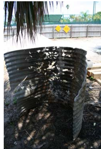
Old Corrugated Metal Pipe
