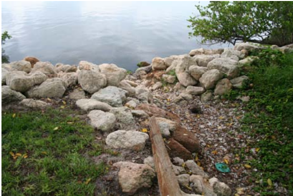
Third Avenue Outfall
