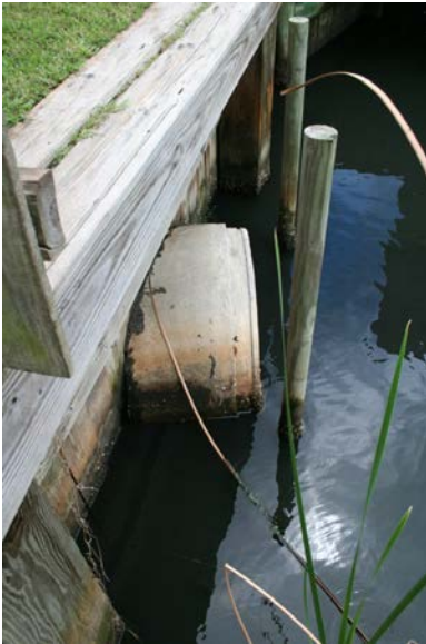
Photo 10 Typical Canal Outfall
