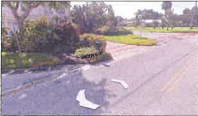
EAST IMAGE - 01 - LOOKING SOUTH
